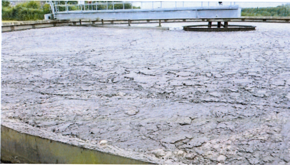
Photograph 1: Thick foam observed on clarifier no. 1.
